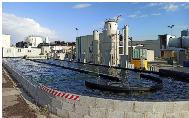
Finished construction of the pilot plants for biogas upgrading in Zaragoza
